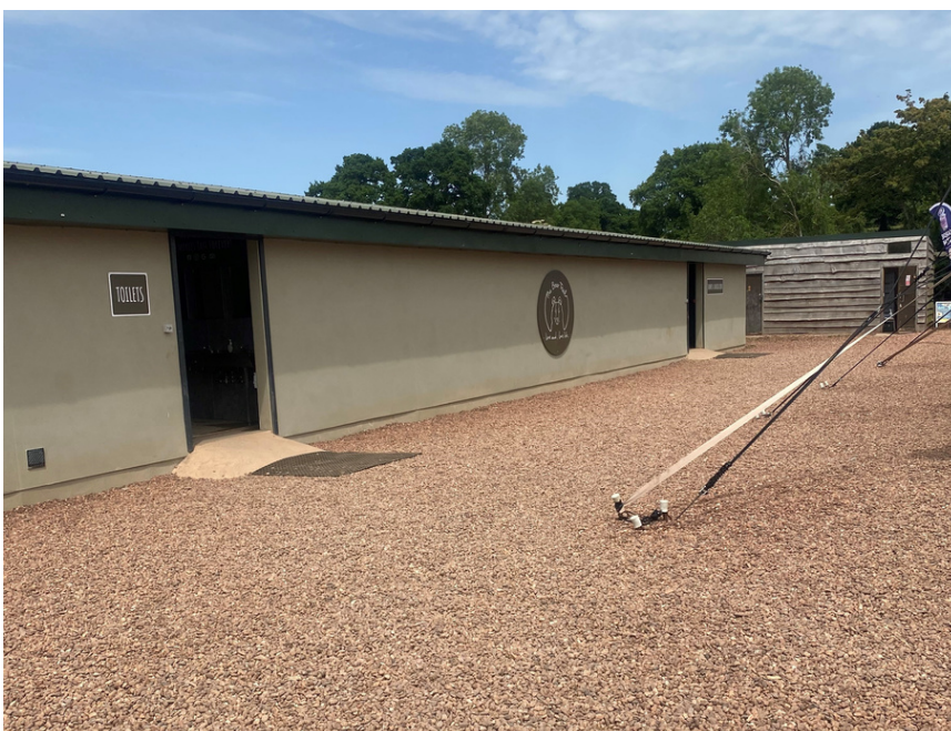
Access To Amenities Block Terrain
